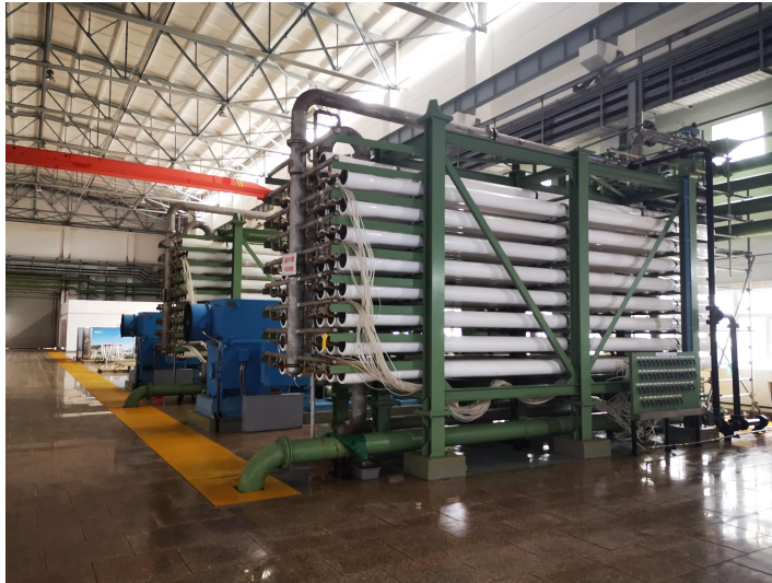
Seawater Desalination System of Sanmen Nuclear Power Plant
